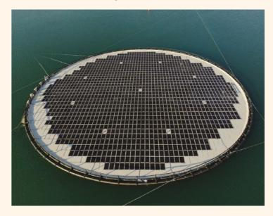
Keppel Infrastructure was awarded a grant from the Energy Market Authority (EMA) and JTC to pilot Singapore's first membrane-based nearshore floating solar photovoltaic (PV) system at Jurong Island. The pilot PV system consists of three circular platforms, which will have an installed capacity of 1.5 MWp.
