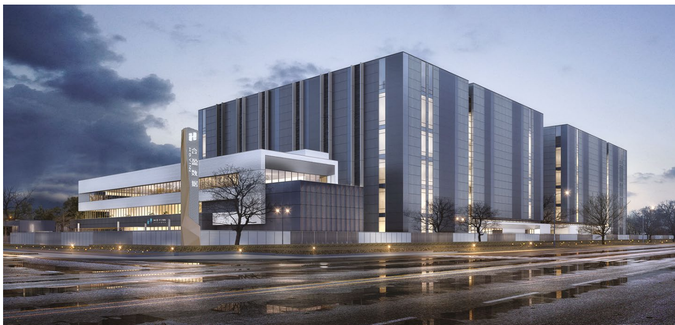
KDC Fund II entered a strategic partnership with Heying, a wholly-owned subsidiary of Tianjin Zhengxin Group, to jointly develop Huailai Data Centre, a greenfield data centre in Greater Beijing.
